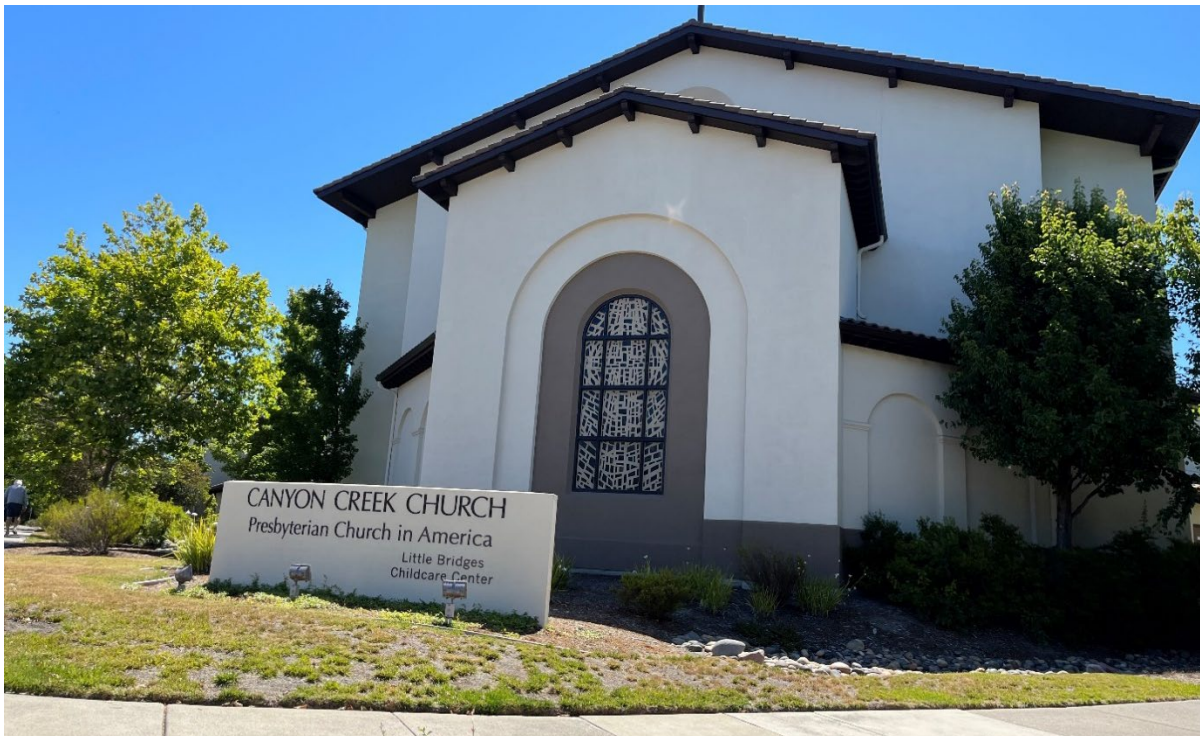
Figure 3.1-8 View 6: Looking southeast toward Canyon Creek Presbyterian Church from intersection of Gale Ridge Road and Bollinger Canyon Road
