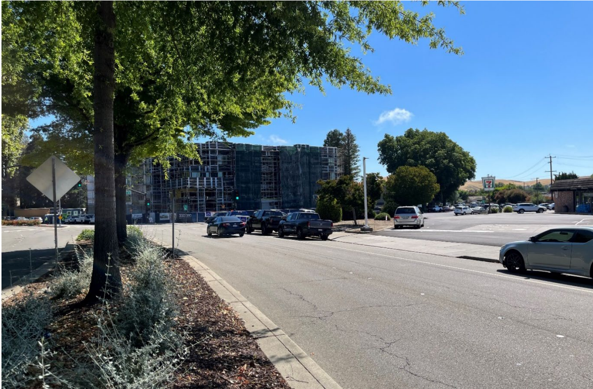
Figure 3.1-3 View 1: Looking northeast toward Aspenwood Apartments from corner of Alcosta Boulevard and Kimball Avenue
