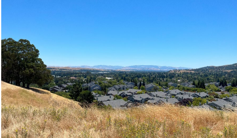
Photograph 2. Photograph of hillside multi-family residential units from the Preserve Residents Clubhouse, looking south-southeast
